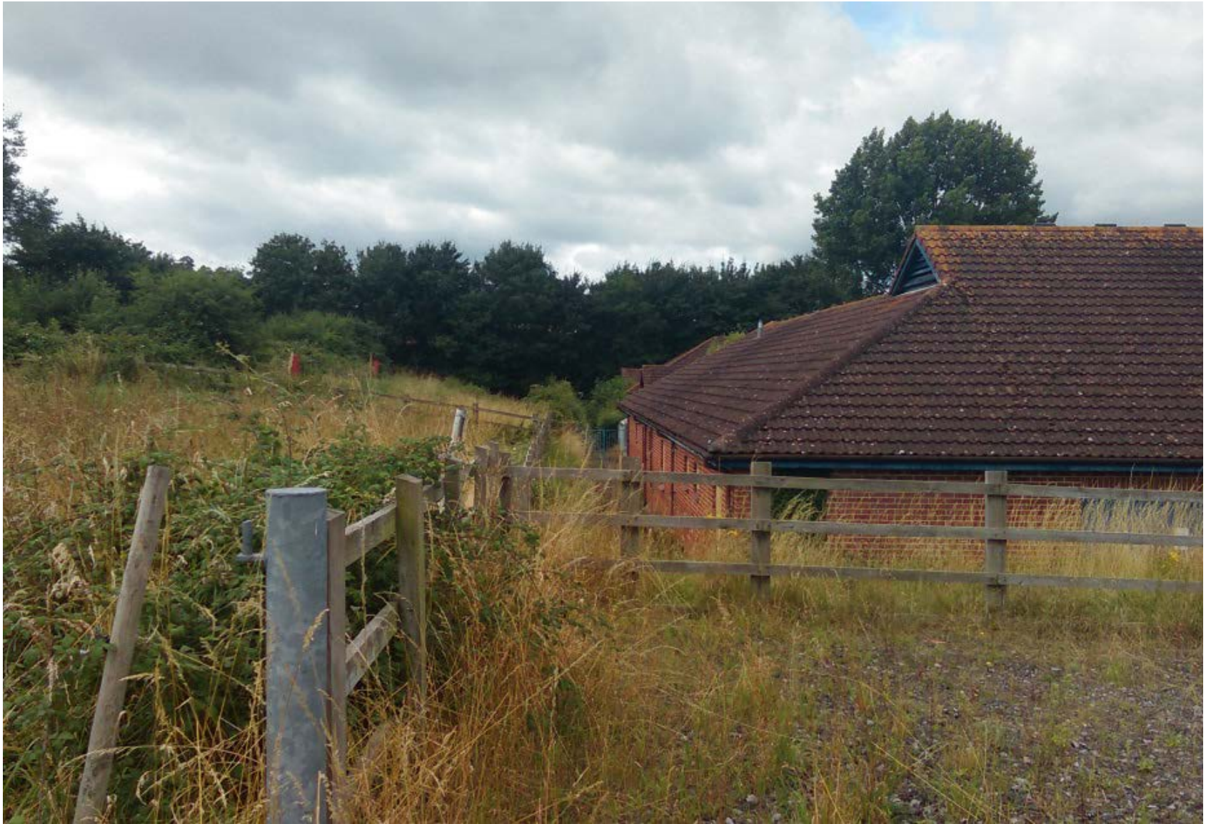
Hospital with pond in background
